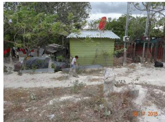
Image 15: A child in MB plays near exposed livewires and an open meter box. Many meter boxes in MB are within reach of pedestrians.
